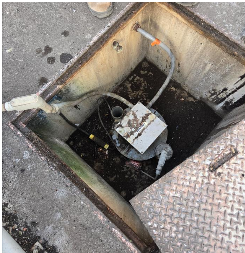
Figure 25: Stilling Well – Water level Sensor Metritape
