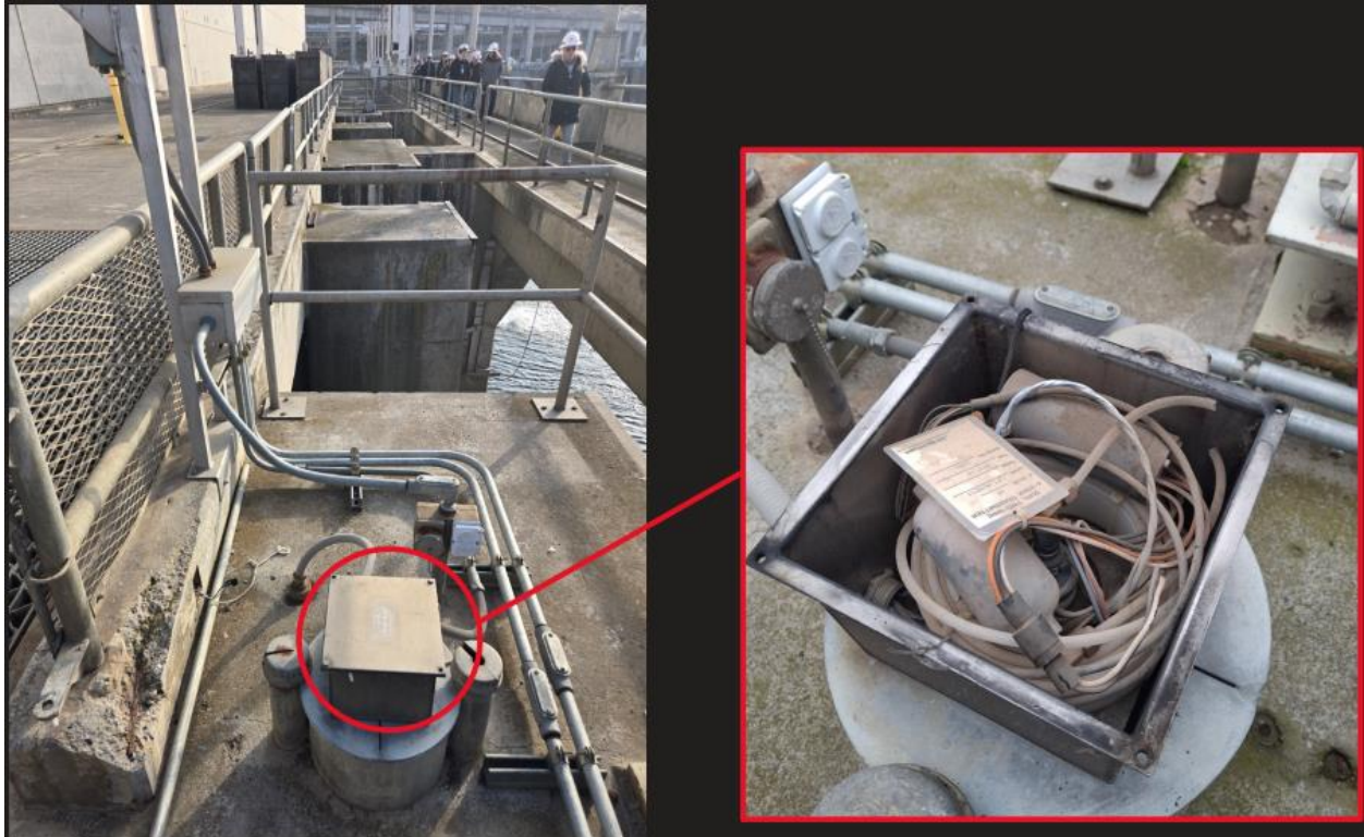
Figure 18: Stilling Well – Water level Sensor Metritape
